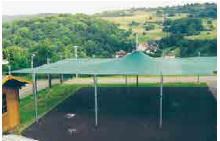
Sun protection covering an outside area at a kindergarten approx. 15.00 x 11.00 m (by Groh)
